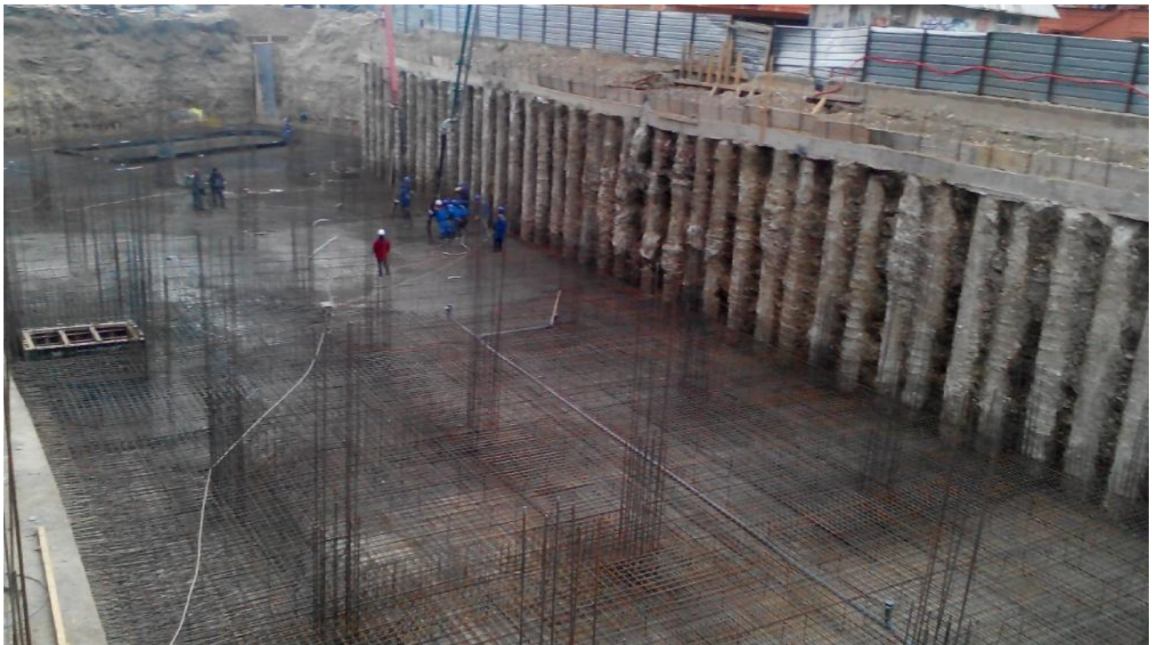
Fig.8 Characteristic photography of the excavated pit
