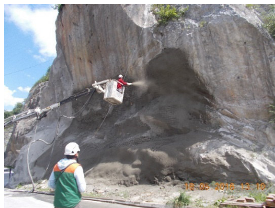
Figure 11. Illustration of phase of application of slope protection measures for Slope Protection Type 3
