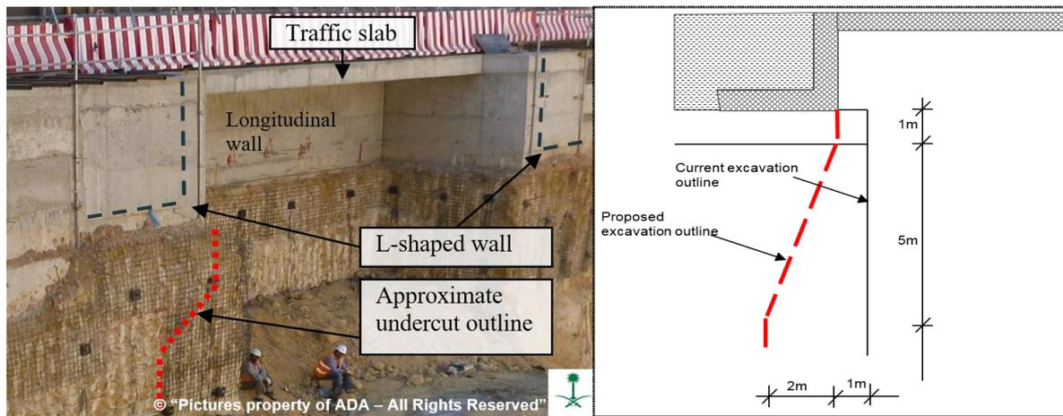
Figure 1: Proposed undercut profile and its dimensions
